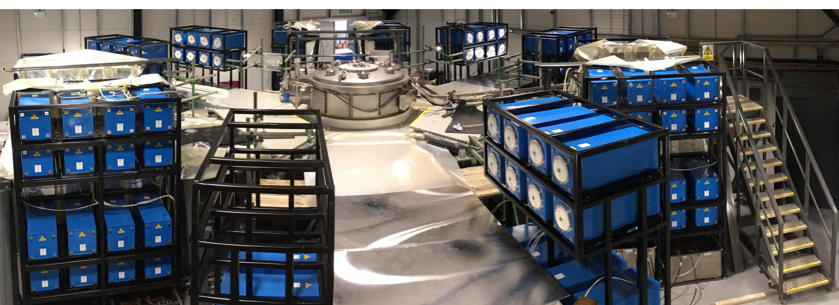
Fig. 4: Panorama of M3 during construction
